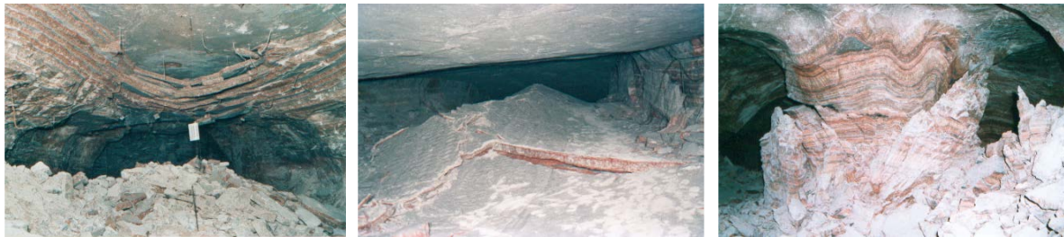
Figure 1: Examples of potential damage due to rock pressure and contour fracturing in underground potash mining
