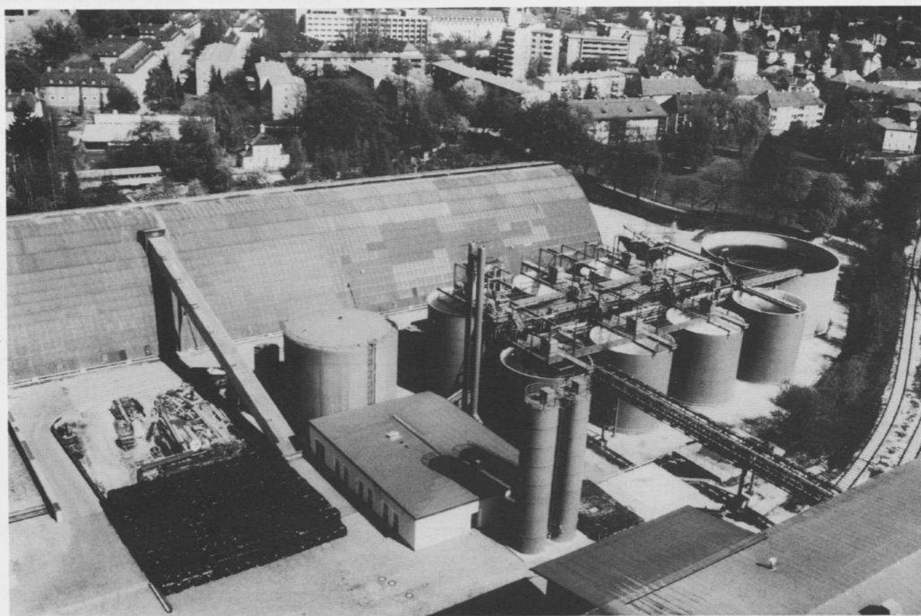
Fig. 6. View of the brine purification plant.
