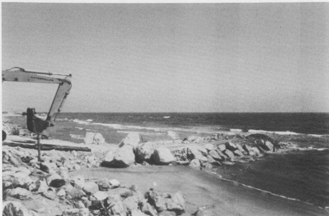
Fig. 3. Sea jetty: creating the core and the "terraccette".
