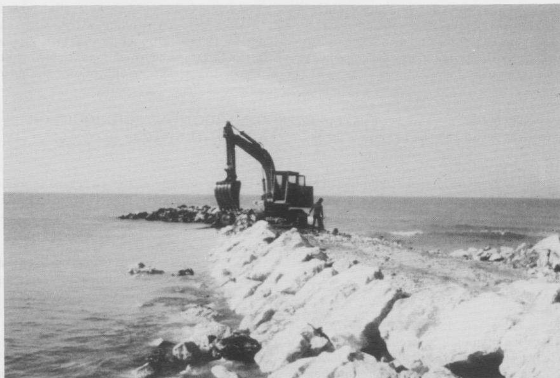
Fig. 4. Sea jetty: creating the shell.
