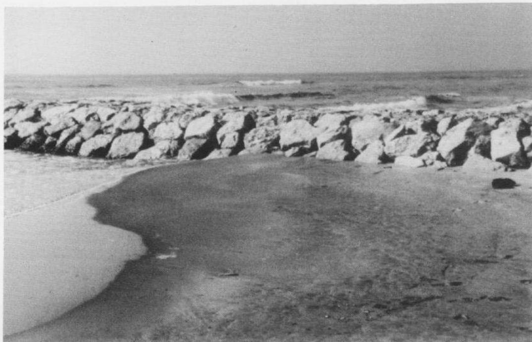
Fig. 5. Sea jetty: upper part of the shell.
